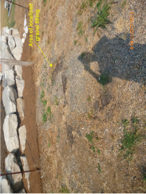
Plate 4: Close up of localised filling along the southern site boundary adjacent to recently constructed residential dwellings. (21/10/2013)
